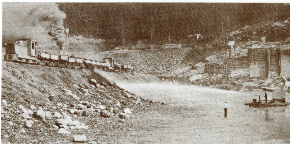
Conklingville Dam under construction
